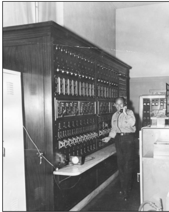
Photo 8: Control & Instrument Room (Haggin Museum)
