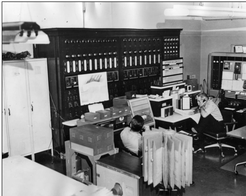
Photo 9: Control and Instrument Room (Haggin Museum)
